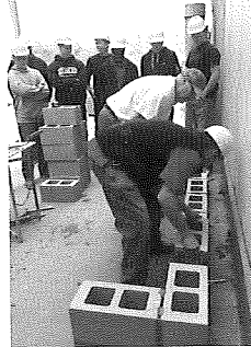
Dunwoody Institute students participate in hands-on experience setting concrete masonry units.
